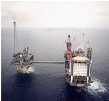
CCS is currently occurring in Norway: CO 2 removed from gas at the Sleipner field and stored deeper underground in a saline aquifer (copyright Statoil)
